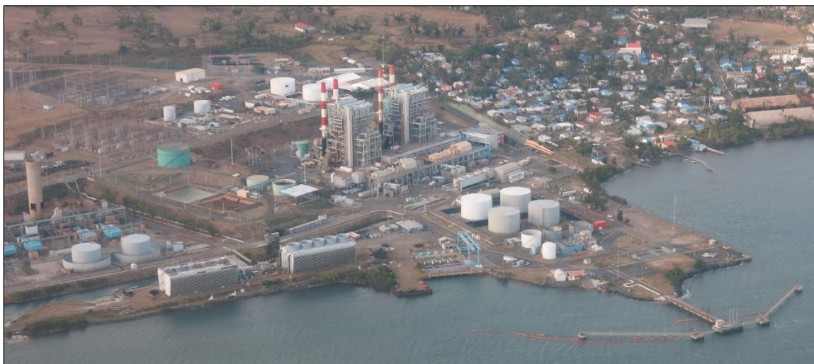
Figure 1. PREPA Aguirre Power Generation Complex, February 2018
