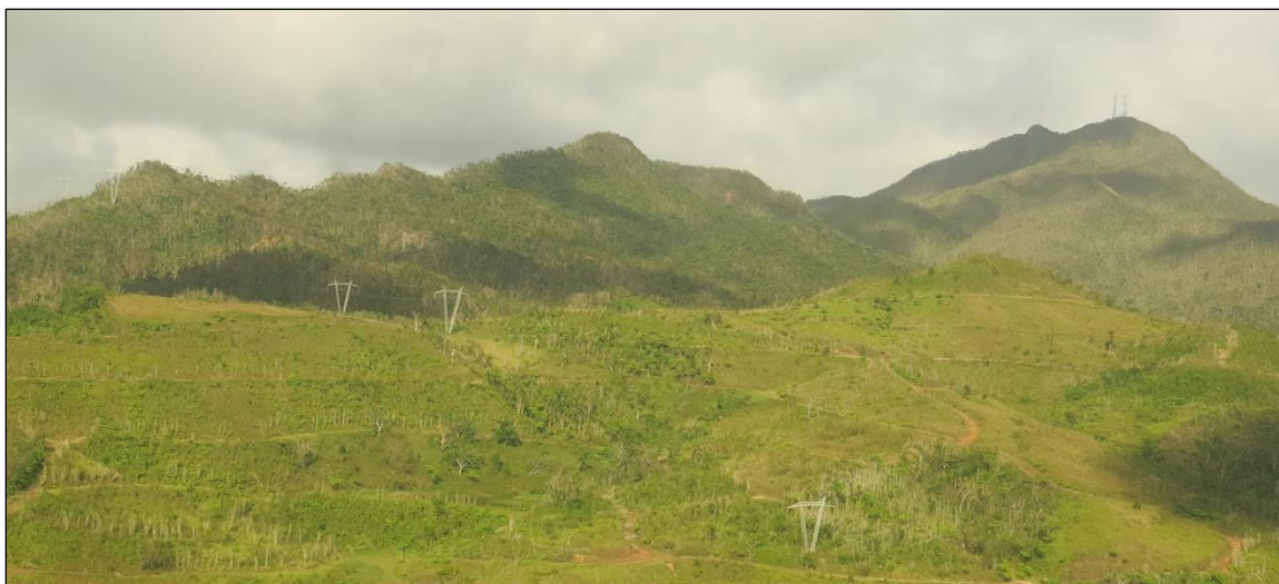
Figure 2. Power Distribution Line in Mountains Southeast of Utuado, Puerto Rico, February 2018
