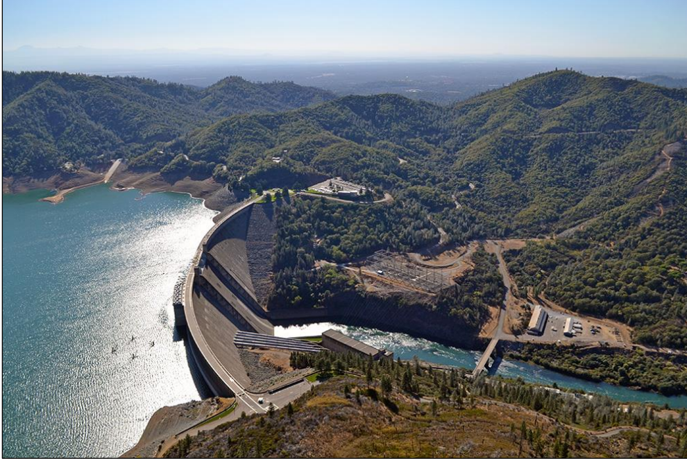
Figure 2. Shasta Dam and Reservoir
