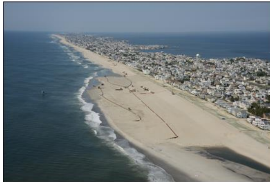
Figure 4. Example of a Beach Engineered to Reduce Flood Damages (Long Beach Island, NJ)
