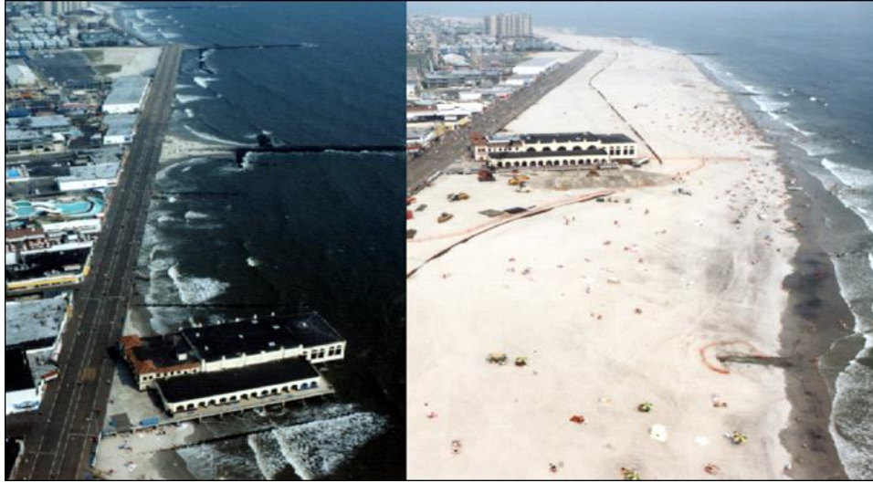
Figure 5. Example of Beach Engineered to Reduce Flood Damages (Ocean City, NJ, before and after engineered beach project)
