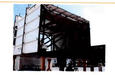
Example of Temporary Bracing Required During Erection Due to Thin Scantling
