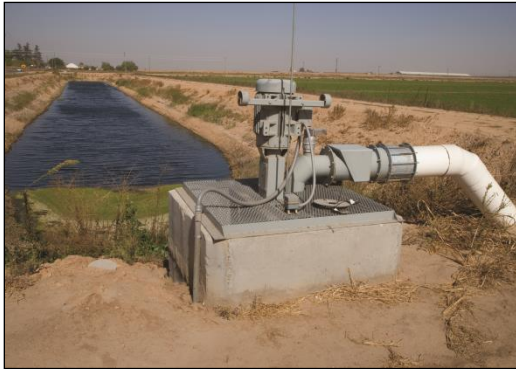
Figure 12. Tailwater Recovery and Pump
