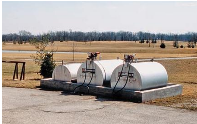
Figure 1. Illustrative Example of Oil Storage Units
