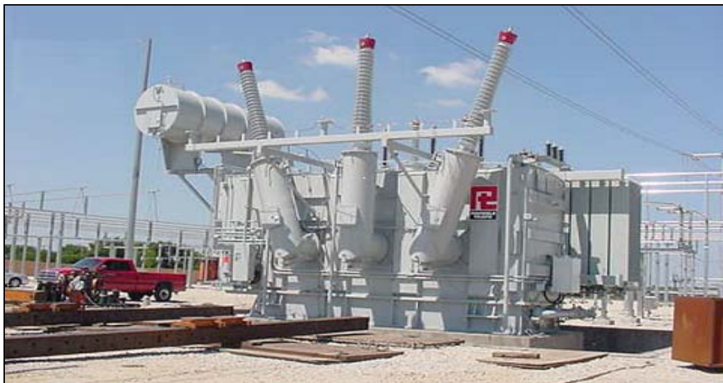
Figure 3. Installation of a 345 kV Transformer
