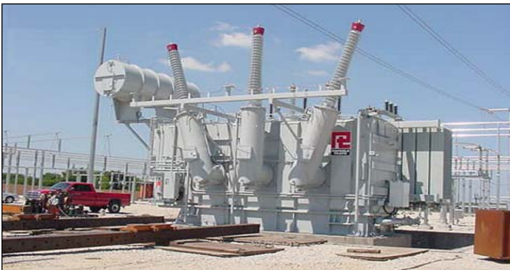
Figure 3. 345 kV Transformer Installation
