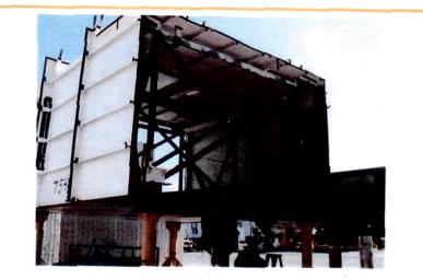
Example of Temporary Bracing Required During Erection Due to Thin Scantling
