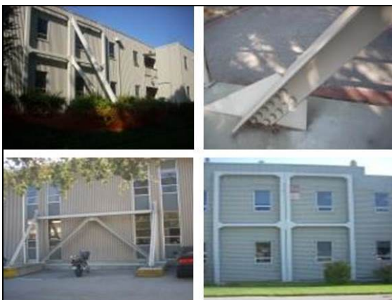
Figure 13. Seismic Bracing of Office Buildings
