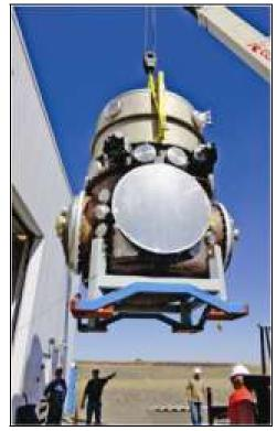
**Source:** National Science Foundation, 2012 NSF Facility Plan, p. 22. **Note:** Movement of end-test mass vacuum chamber of AdvLigo.
