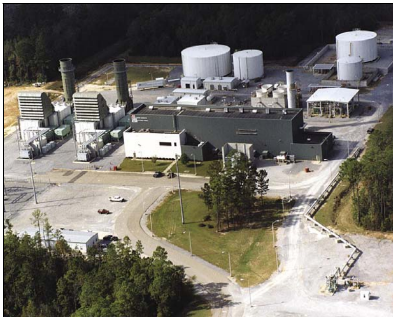
Figure 18. 110 MW CAES Plant in McIntosh, AL
