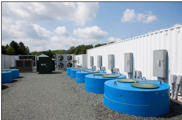
Figure 30. Part of a 1 MW Flywheel System in the ISO-New England Grid
