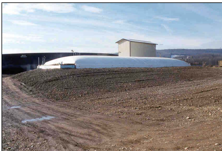
Figure 3. Plug Flow AD System
