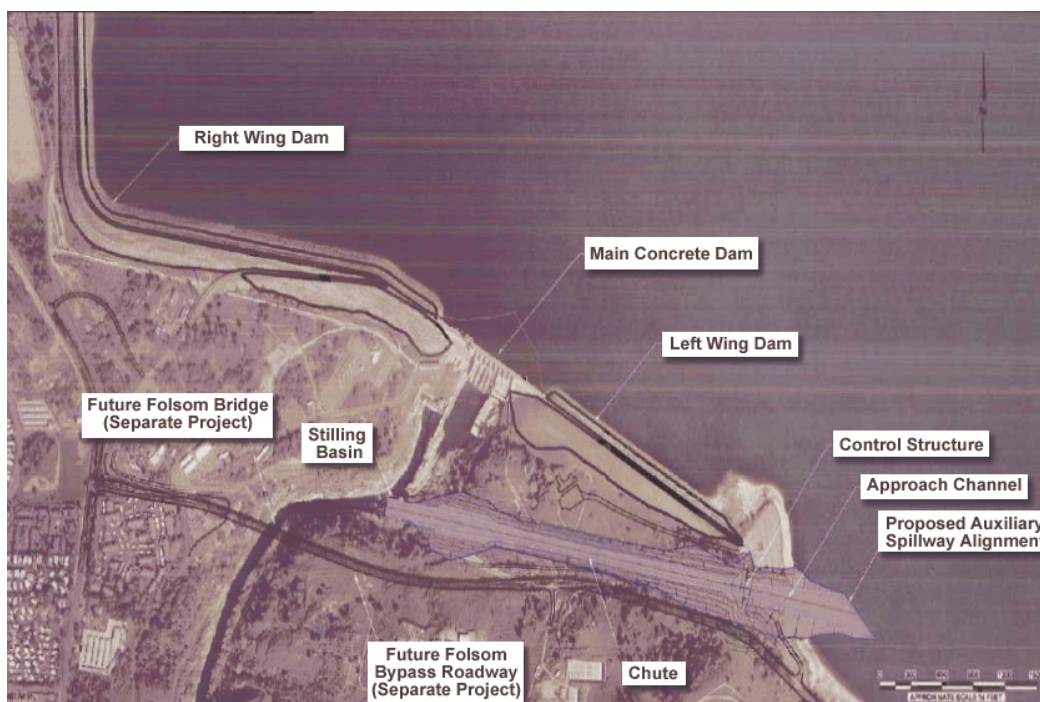
Figure 5. Potential Auxiliary Spillway
